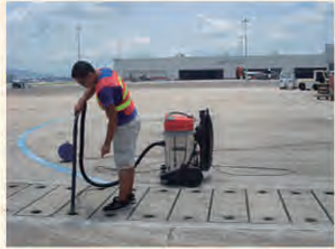
清潔工人正在清理停機坪上的垃圾及碎石。 Workers were clearing debris from airport ramp.
